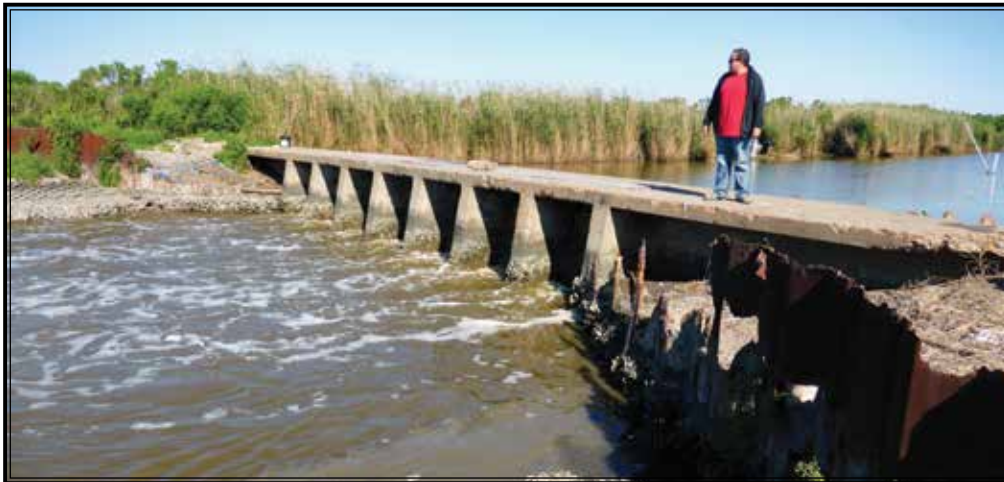
The 55-year-old structure used to manage salinity and water levels in Rockefeller Refuge Unit 4 was failing.
