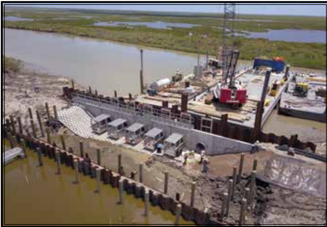
Innovative structure design included use of concrete T-walls that should better withstand the coastal environment and provide better management abilities.
