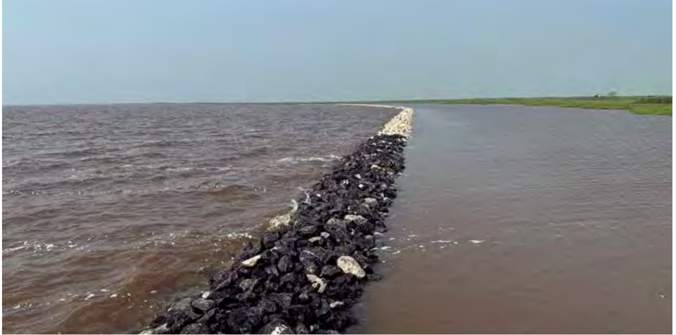
Newly installed breakwater at Anahuac National Wildlife Refuge.
