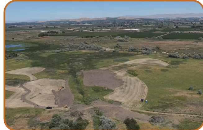
July 2026 - During construction
