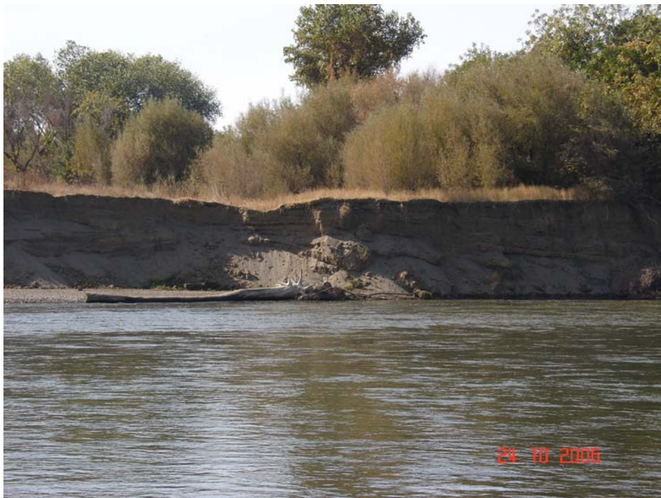
Figure 4. Photograph of the middle part of the downstream part of the site prior to construction of the rock-toe/brush revetment (Photo taken on 10/24/2006).
