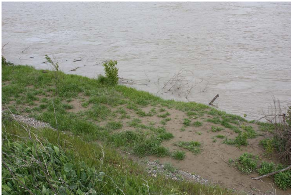
Figure 17. View of the top of submerged woody material that was incorporated into the revetment at about Elevation 117 feet. Flow in the river was about 11,000 cfs (Photo taken on 04/12/2008).
