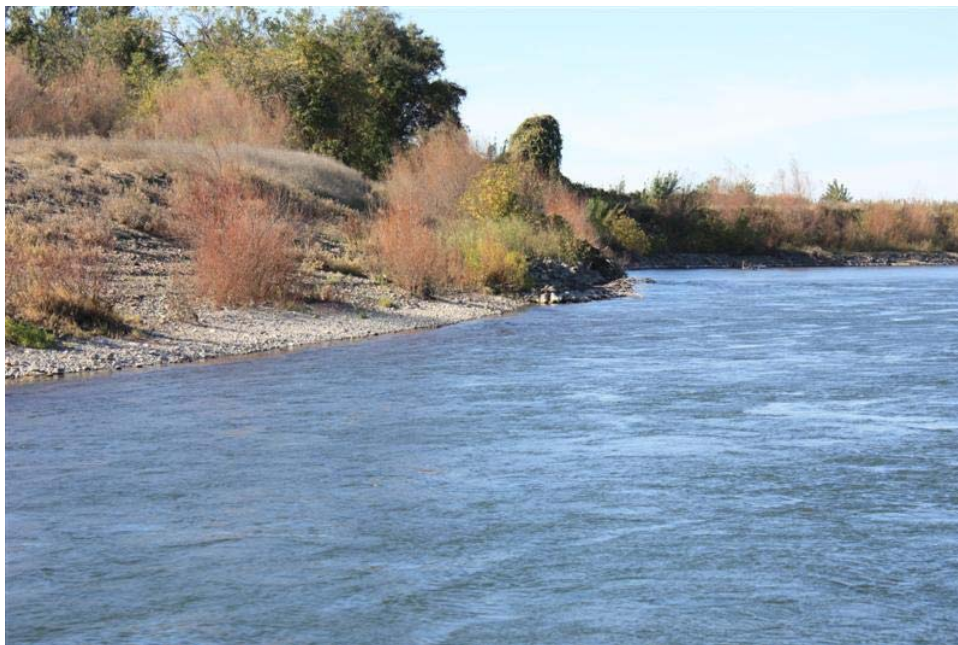
Figure 35. Downstream end of revetment. Note presence of willows growing on the bar which indicates there has been no retreat of the bank downstream of the toe rock.
