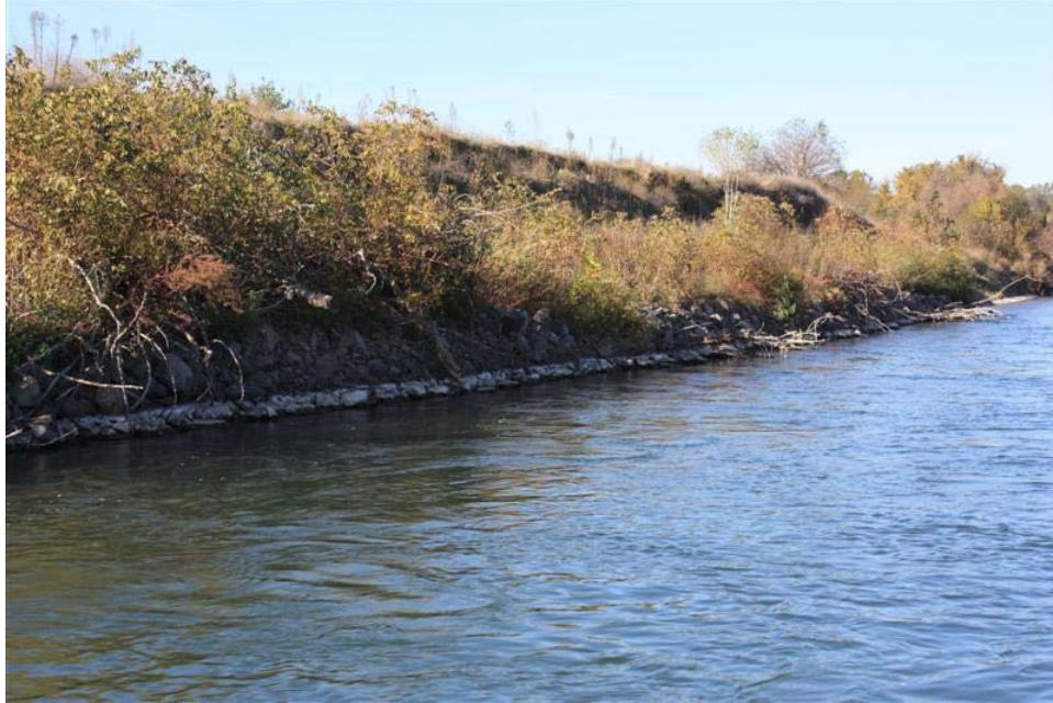
Figure 30. Close up view of the upper section of the toe rock revetment. There is no evidence of loss of rock.
