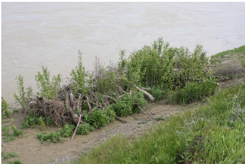
Figure 19. Close up view of a woody debris pile cabled onto the top of the revetment showing volunteer woody plants growing within and around the debris pile. Flow in the river was about 11,000 cfs (Photo taken on 04/12/2010).
