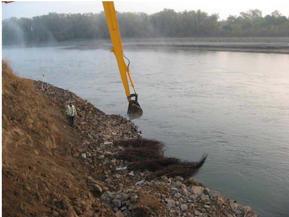
Figure 9. View of woody material being placed on the top of the revetment at about Elevation 119 feet during construction of the revetment (Photo taken on 10/30/2007).
