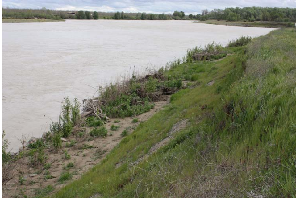
Figure 18. View downstream of the top of the revetment showing the woody debris piles that were placed and cabled onto the revetment. Flow in the river was about 11,000 cfs (Photo taken on 04/12/2008).
