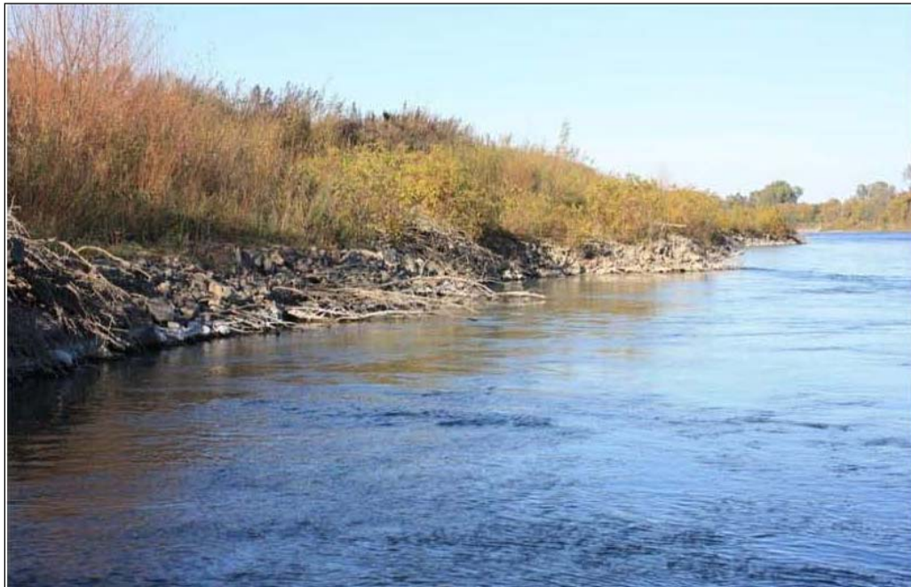
Figure 3.7-4. Upstream View of the Middle Section of the Rock-toe and Tree Revetment Under Existing Conditions. Note the Dense Riparian Vegetation Species Voluntarily Growing on the Top of the Rock, and the Presence of the Emplaced Large Woody Material on the Top of the Rock and within the Revetment (Tetra Tech 2012a).
