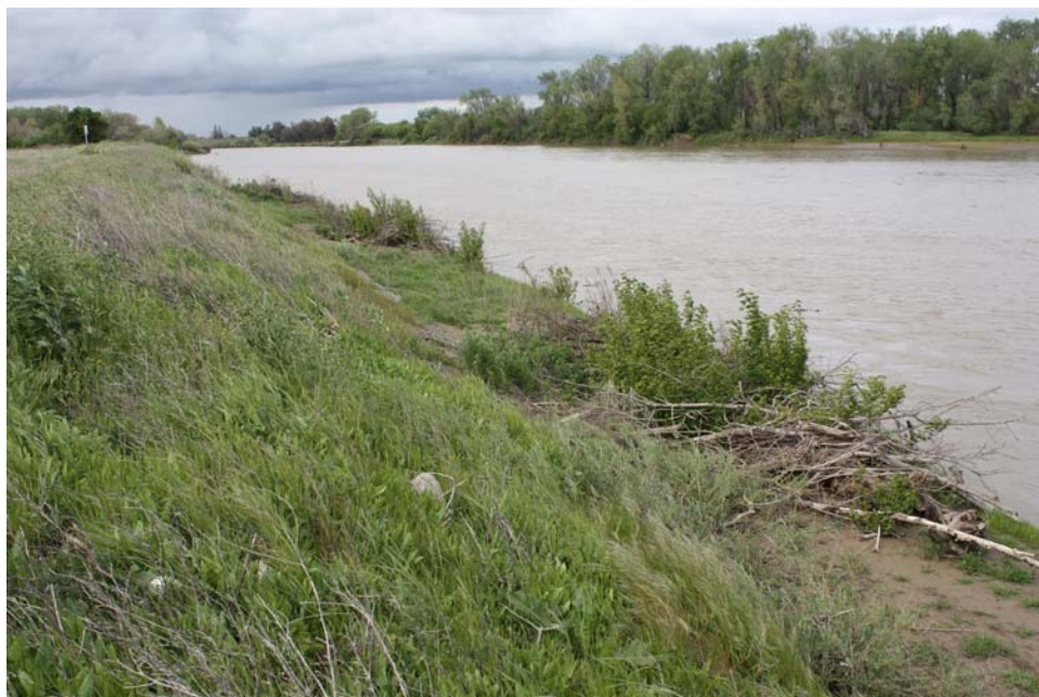
Figure 16. View upstream of the revetment showing the presence of the woody debris piles that were constructed on top of the structure. Flow in the river was about 11,000 cfs (Photo taken on 04/12/2010).
