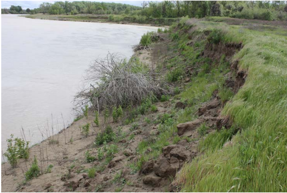
Figure 20. View downstream of eroding upper bank above the top of the revetment that is causing the bank angle to be reduced. Flow in the river was about 11,000 cfs (Photo taken on 04/12/2010).
