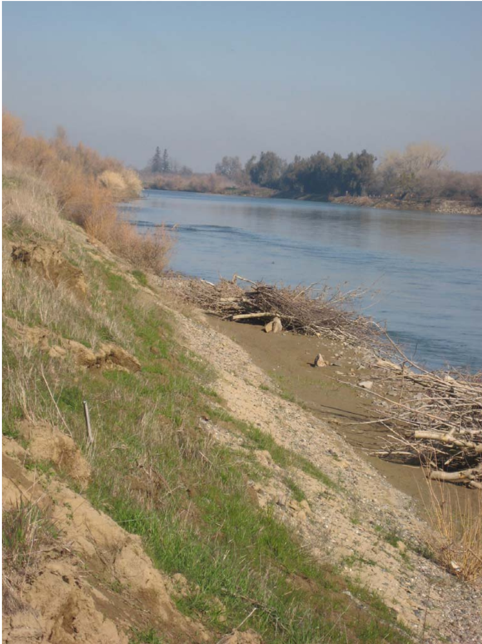
Figure 11. View upstream of the upstream end of the revetment showing the presence of the pre-construction vegetation on the upstream bank (Photo taken on 03/12/2008).
