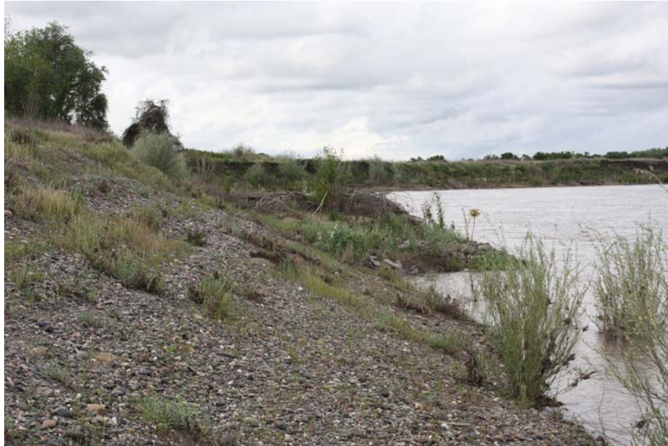
Figure 24. View upstream of the downstream end of the revetment and the downstream tie back. Flow in the river was about 11,000 cfs (Photo taken on 04/12/2010).
