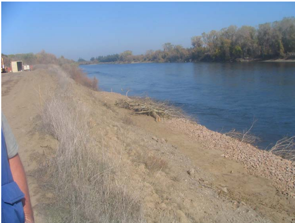
Figure 10. View upstream of backfill in place between the rock revetment and the bank slope during construction (Photo taken 10/30/2007).
