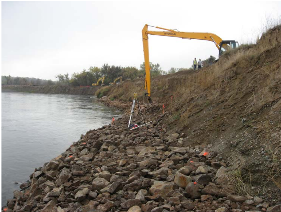
Figure 7. View downstream of the rock toe being emplaced during construction of the revetment. The top of the rock is at Elevation 119 feet (Photo taken on 10/30/2007).
