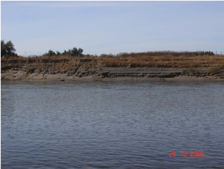
Figure 1. Photograph of the upstream end of the site prior to construction of the rock-toe/brush revetment (Photo taken on 10/24/2006).
