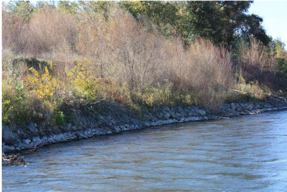
Figure 34. Upstream view of the lower end of the toe rock revetment. Note presence of volunteered riparian vegetation species as well as emplaced large woody debris on the top of the rock and within the rock. There is no evidence of loss of rock from the revetment.
