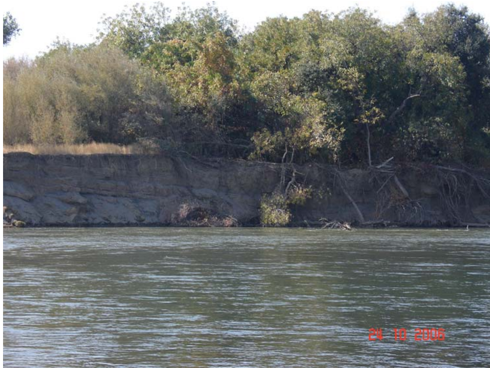
Figure 3. Photograph of the apex of the eroding bend prior to construction of the rock-toe/brush revetment (Photo taken on 10/24/2006).
