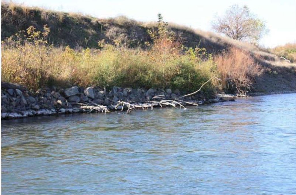
Figure 3.7-3. Upstream View of the Upstream End of the Rock-toe and Tree Revetment Under Existing Conditions. Note: (a) the Presence of Riparian Vegetation as well as the Large Woody Material Emplaced within the Rock During Construction; (b) there is No Evidence of Loss of Rock; and (c) the Larger Anchor Boulders used to Secure the Large Woody Material Emplaced on the Top of the Revetment (Tetra Tech 2012a).
