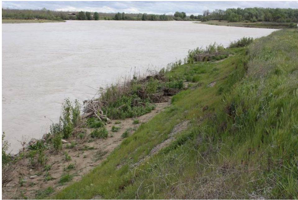
Figure 18. View downstream of the top of the revetment showing the woody debris piles that were placed and cabled onto the revetment. Flow in the river was about 11,000 cfs (Photo taken on 04/12/2010).
