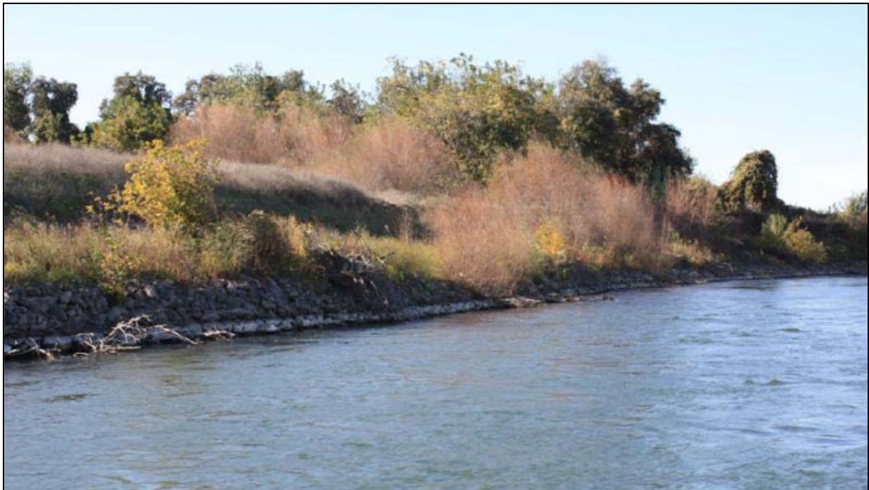
Figure 3.3-2. Upstream View of the Lower (Downstream) End of the Rock-toe and Tree Revetment. In Addition to the Embedded Tree Clusters, Note the Presence of Volunteered Riparian Vegetation Species Including Sycamore, Box Elder and Willows on the Ssurface of the Rock (Source: Tetra Tech 2012a).
