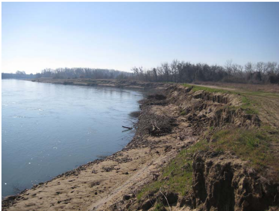
Figure 13. View downstream of bank erosion caused by the first higher winter flows after construction (Photo taken on 03/12/2008).
