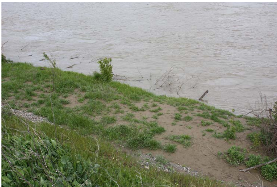
Figure 17. View of the top of submerged woody material that was incorporated into the revetment at about Elevation 117 feet. Flow in the river was about 11,000 cfs (Photo taken on 04/12/2008).
