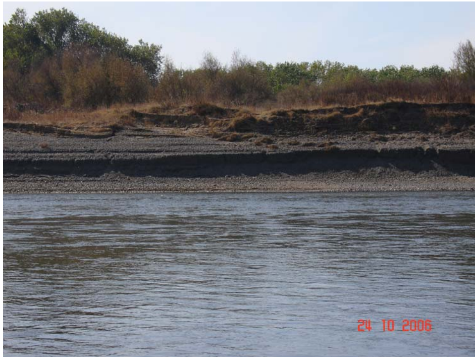
Figure 5. Photograph of the downstream end of the site prior to construction of the rock-toe/brush revetment (Photo taken on 10/24/2006).
