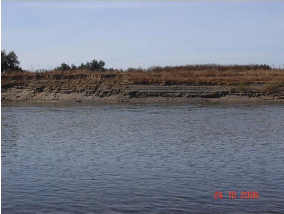
Figure 1. Photograph of the upstream end of the site prior to construction of the rock-toe/brush revetment (Photo taken on 10/24/2006).
