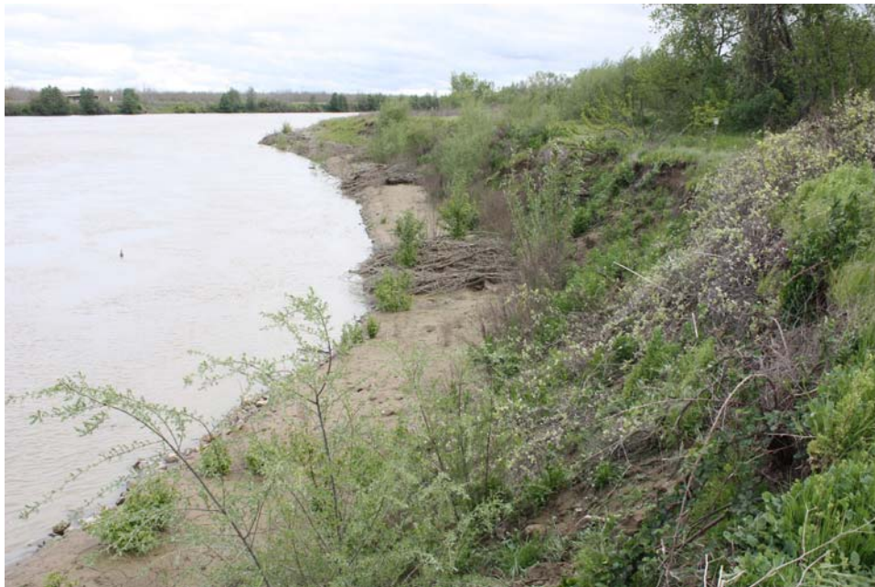
Figure 23. View downstream of the downstream part of the revetment with vegetation growing at the toe of the bank and on the top of the revetment. Flow in the river was about 11,000 cfs (Photo taken on 04/12/2010).
