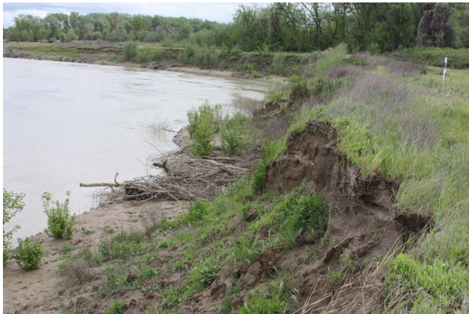
Figure 21. View downstream showing eroding upper bank but no evidence of any scour of the backfill material at the base of the bank. Flow in the river was about 11,000 cfs (Photo taken on 04/12/2008).
