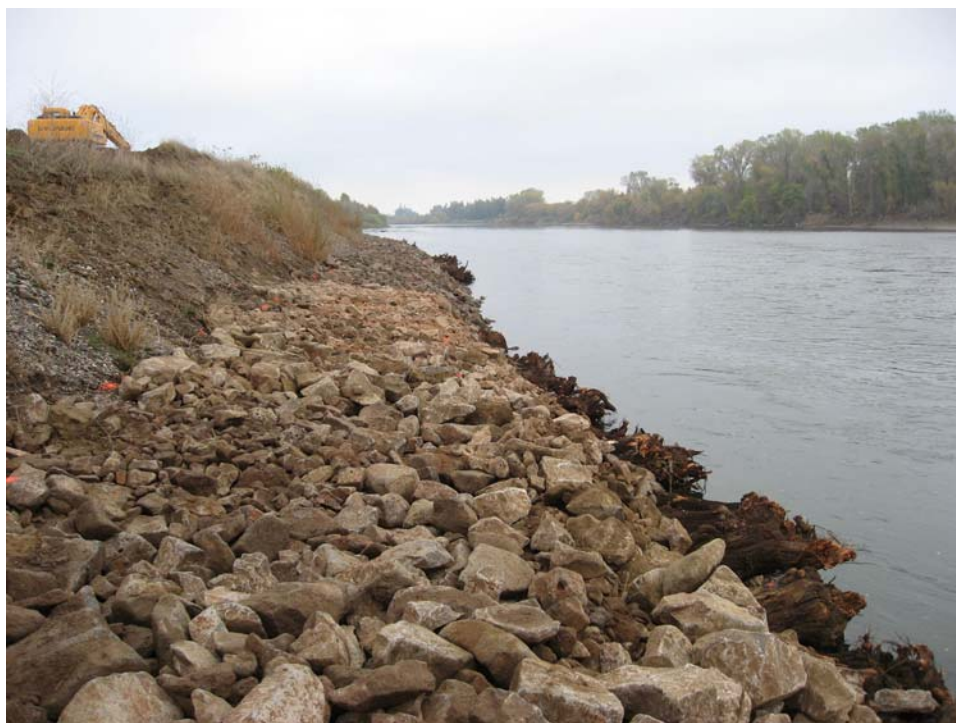
Figure 8. View upstream of the rock toe being emplaced during construction of the revetment. Note the woody material incorporated into the revetment at about Elevation 117 feet (Photo taken on 10/30/2007).
