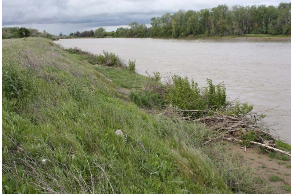
Figure 16. View upstream of the revetment showing the presence of the woody debris piles that were constructed on top of the structure. Flow in the river was about 11,000 cfs (Photo taken on 04/12/2010).
