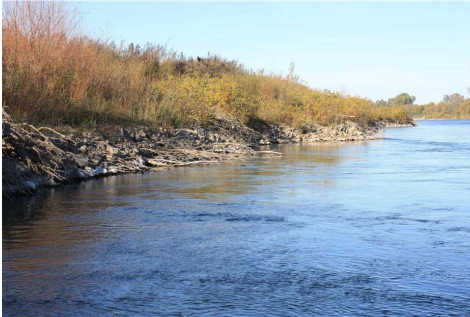
Figure 32. Upstream view of the middle section of the toe rock revetment. Note the very dense volunteered riparian vegetation species growing on the top of the rock and the presence of the emplaced large woody debris on the top of the rock and within the rock.
