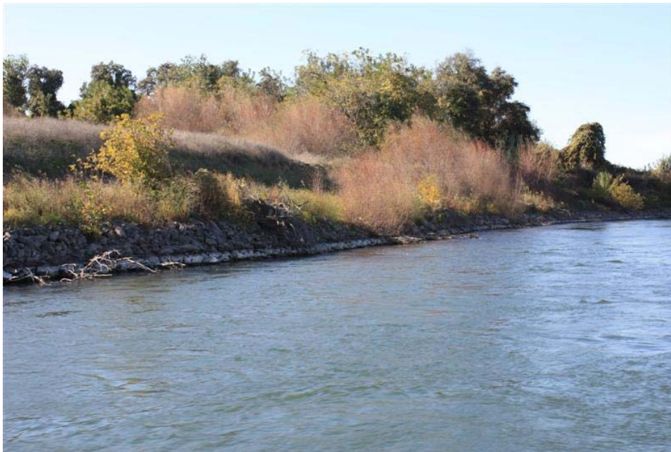
Figure 32. Upstream view of the middle section of the toe rock revetment. Note the very dense volunteered riparian vegetation species growing on the top of the rock and the presence of the emplaced large woody debris on the top of the rock and within the rock.
