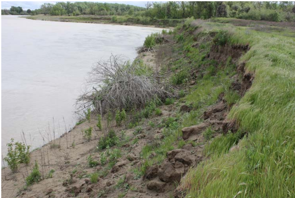
Figure 20. View downstream of eroding upper bank above the top of the revetment that is causing the bank angle to be reduced. Flow in the river was about 11,000 cfs (Photo taken on 04/12/2010).
