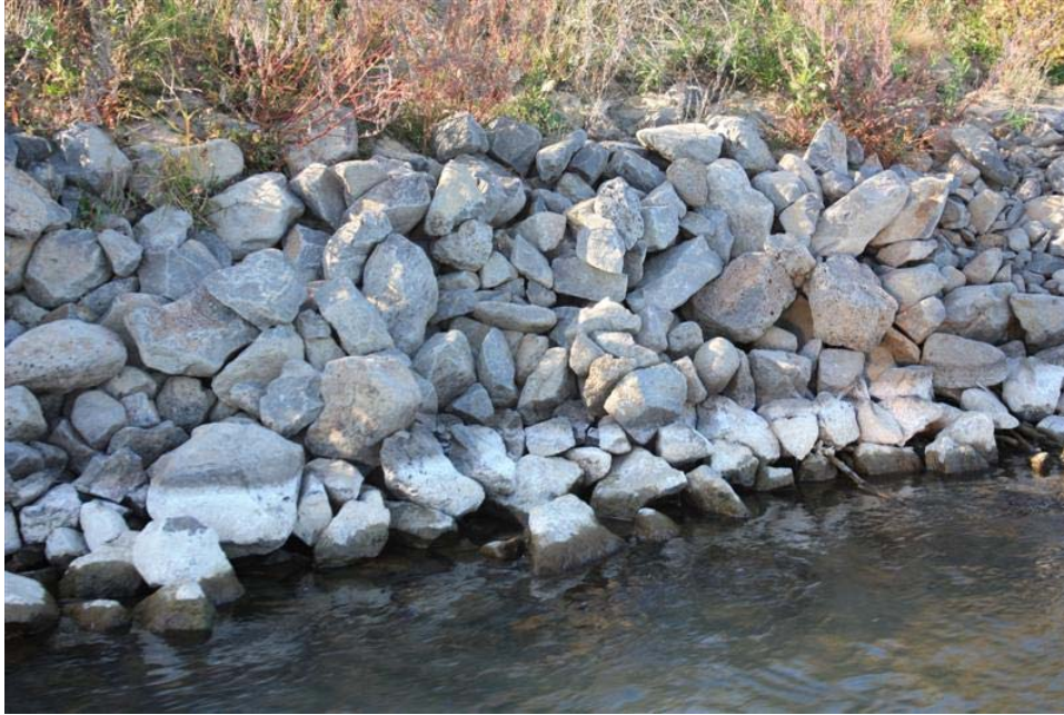
Figure 28. Close up view of the rock toe within the middle section of the revetment. There is no evidence of loss of rock.
