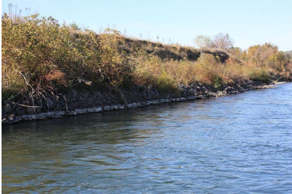
Figure 30. Close up view of the upper section of the toe rock revetment. There is no evidence of loss of rock.
