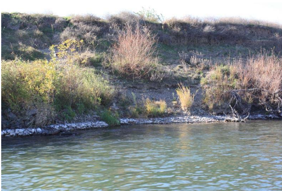
Figure 25. View of the upstream end of the rock revetment and transition to unprotected bank. Note the presence of the willows growing on the bank indicating that there has been little or no erosion at the upstream end of the revetment.
