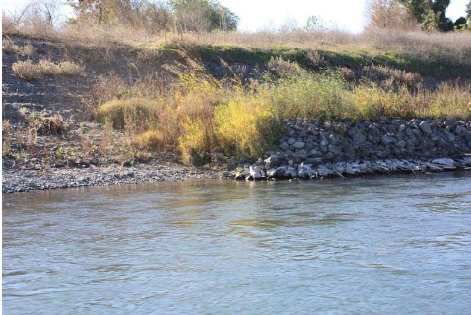
Figure 36. Close up view of the downstream end of the toe rock. Rock is intact and there appears to be little loss of rock at the downstream end.
