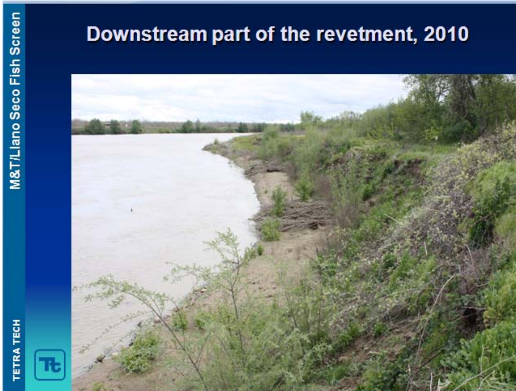
This slide shows the downstream end of the revetment with reasonable revegetation being recruited at the site.
