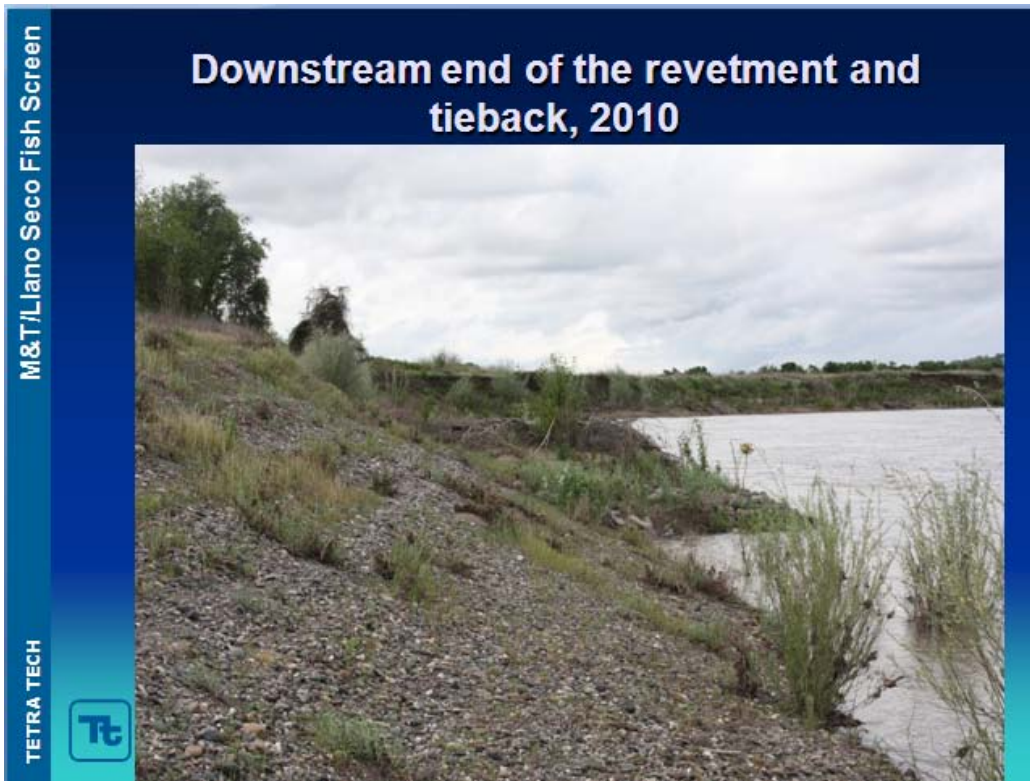
This slide shows the end of the structure with no retreat of the bank. The willows downstream are a reasonable marker.
