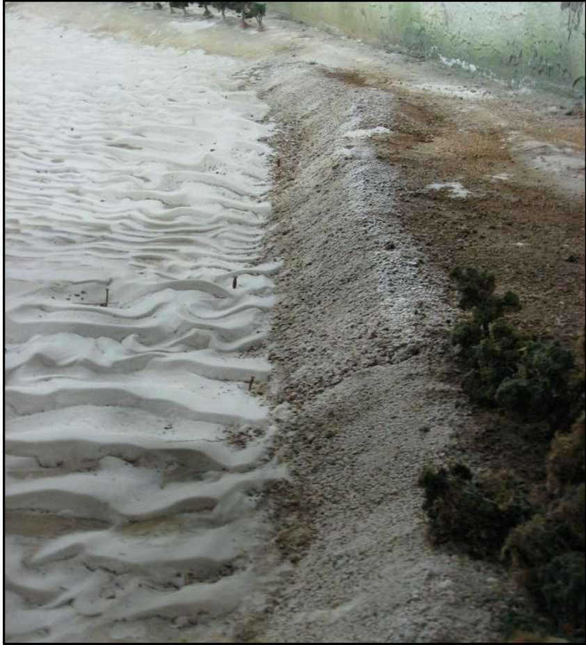
Figure 2-12: Realigned east bank.
