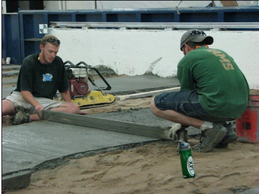
Figure 2-5: Construction and leveling of concrete cap.
