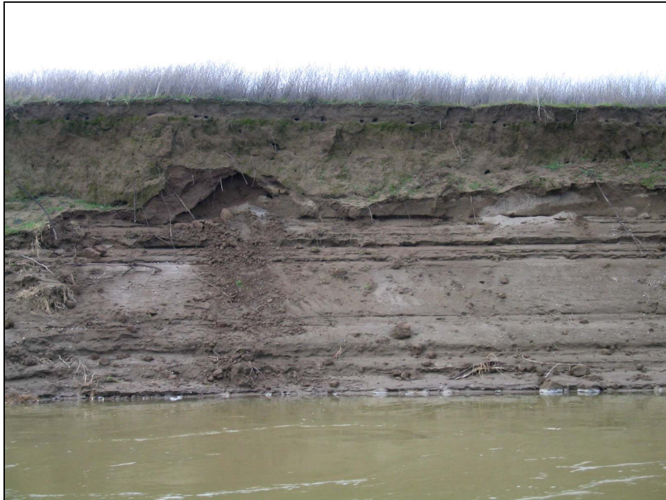
Figure 4. View of the eroding right bank of the Sacramento River at RM 193.
