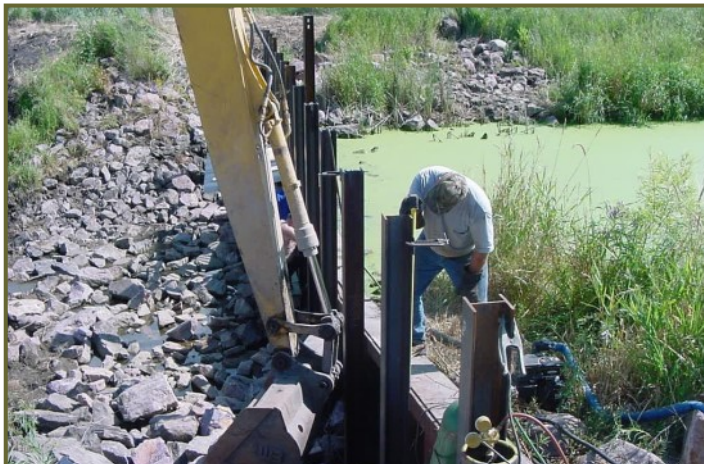
Above: The work on the mechanical fish barrier included adding vertical I-beams to attach the horizontal bars, screens, and catwalk across the top of the structure.
