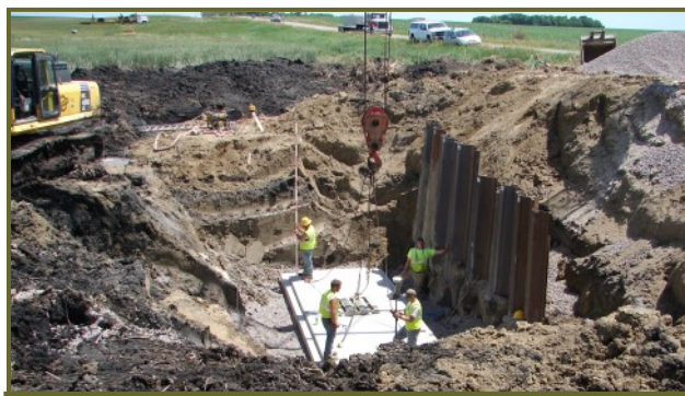
Above: Construction begins on the control structure along County Highway 26 for the Upper Lightning Lake outlet.
