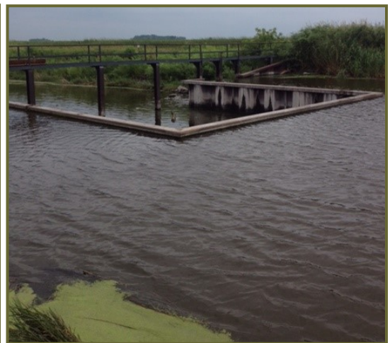
Above: A downstream view of the upper structure shows the large size of the 90-foot weir crest and the 60-foot catwalk across the downstream ditch.
