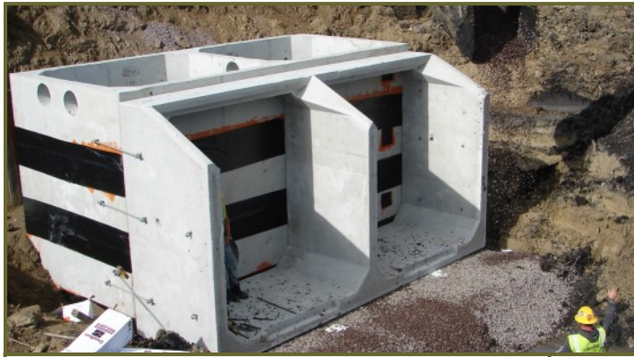
Above: The two bay inlet structure being installed. Note the worker in the inlet area on the left for scale.
