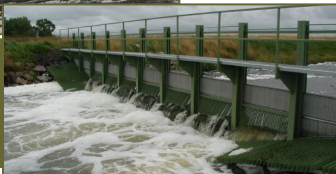
Above: The work on the mechanical fish barrier included adding vertical I-beams to attach the horizontal bars, screens, and catwalk across the top of the structure.
